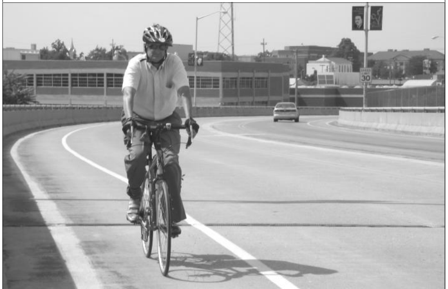
Public Works has restriped Benton/Kimbrough Ave., south of Chestnut Expressway, to merge 4 skinny lanes into 2 — and included bike lanes. What a great solution!
