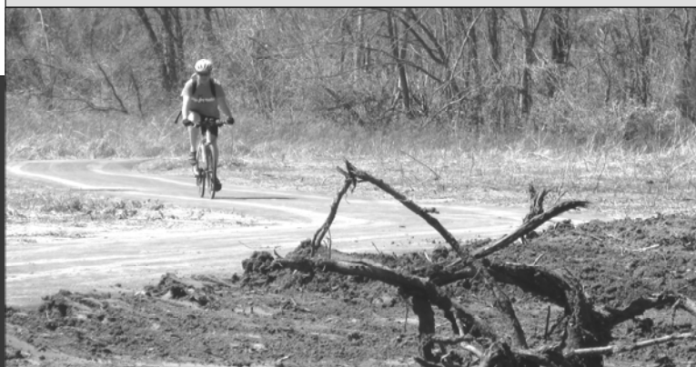
Evidence of the ongoing 60/65 highway interchange construction will continue to be visible from Galloway Creek Greenway until 2012.
